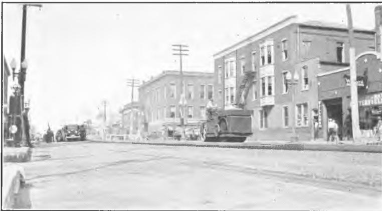
Fig. 5. U. S. Route 12 through Michigan City. Resurfacing old brick pavement with a binder course of asphaltic concrete and a wearing course of rock asphalt.
