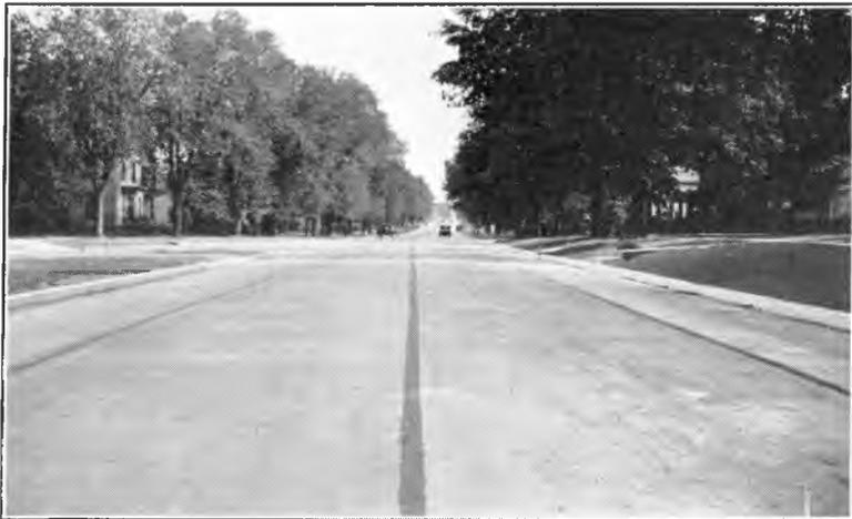
Fig. 4. State Route 55 through Crown Point. Looking southward from station 22+00 after removal of car tracks and construction of 36-foot reinforced concrete pavement.
