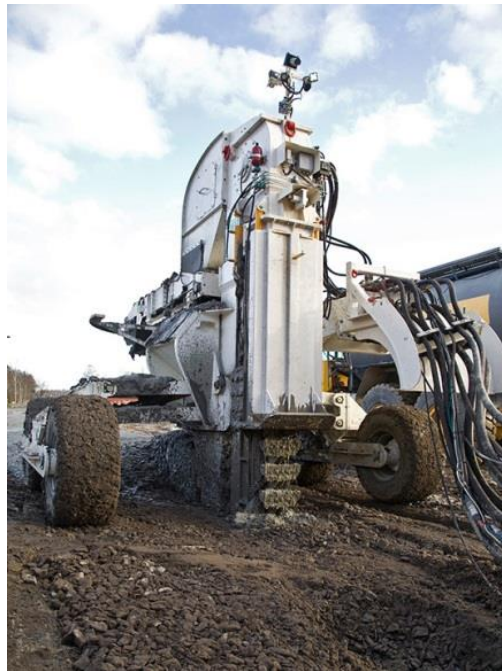
FIGURE 4 PIPE EXPRESS® OPERATION IN SWAMPY AREA IN STOCKHOLM, SWEDEN
