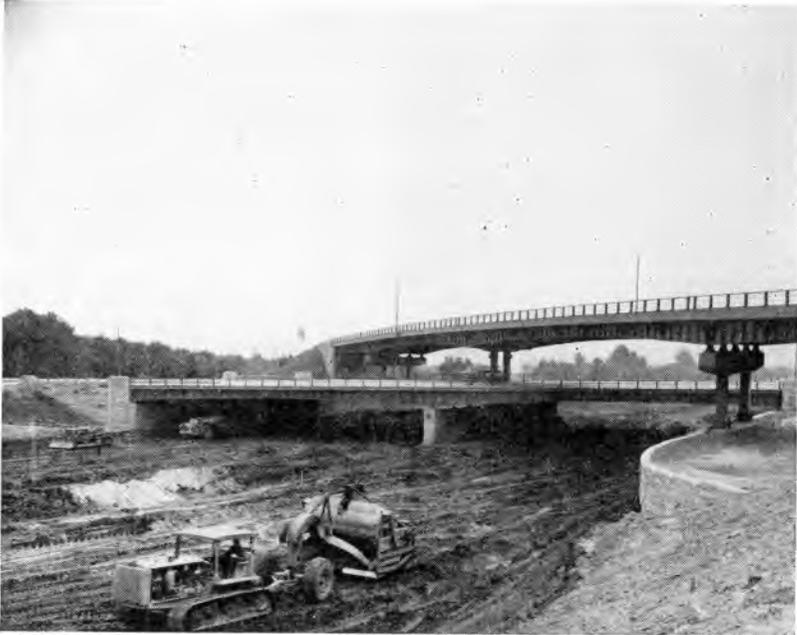
Figure 5. At a point in Woodbridge Township, the Turnpike passes under two existing highways. The upper route is Woodbridge Avenue, the middle level is Route 4 Parkway. Equipment is shown completing excavation for the lower Turnpike level.
