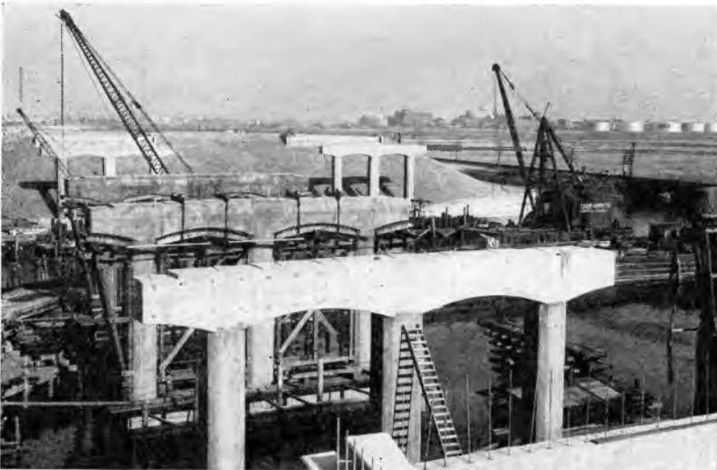
Figure 3. Construction of substructures for the Rahway River crossing. This dual crossing provides two separate parallel structures, one for northbound traffic and the other for southbound traffic. Both will be identical in size and design.
