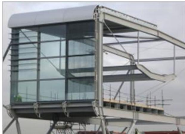
FIGURE 2 EXAMPLE OF CONX SPACE FRAME SYSTEM
