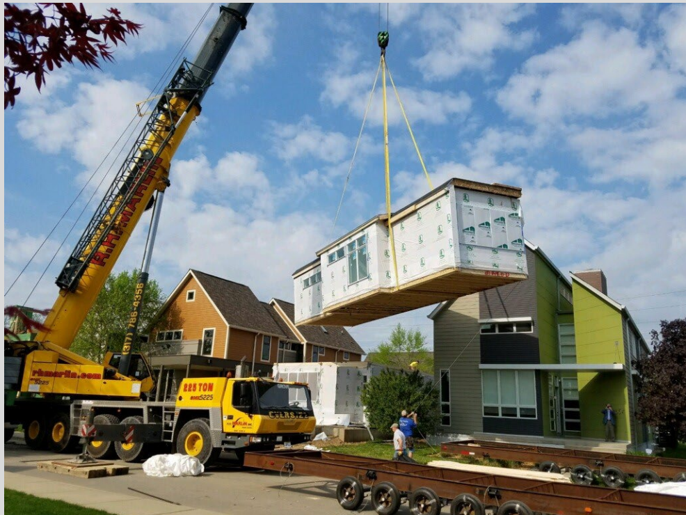
Assembling Modular Homes (photo credits: Indy Mod Homes)
