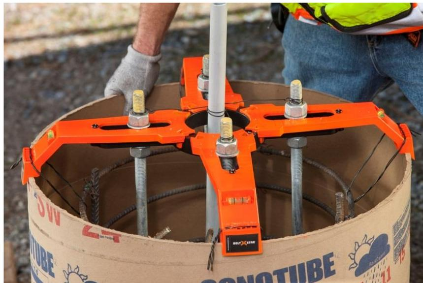
FIGURE 1 BOLT STAR INSTALLED ON FORMING TUBE
