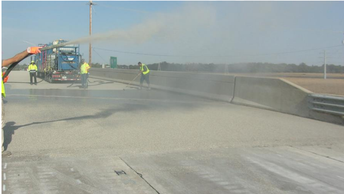
Polymeric bridge deck overlay on westbound I-74 over SR 44
