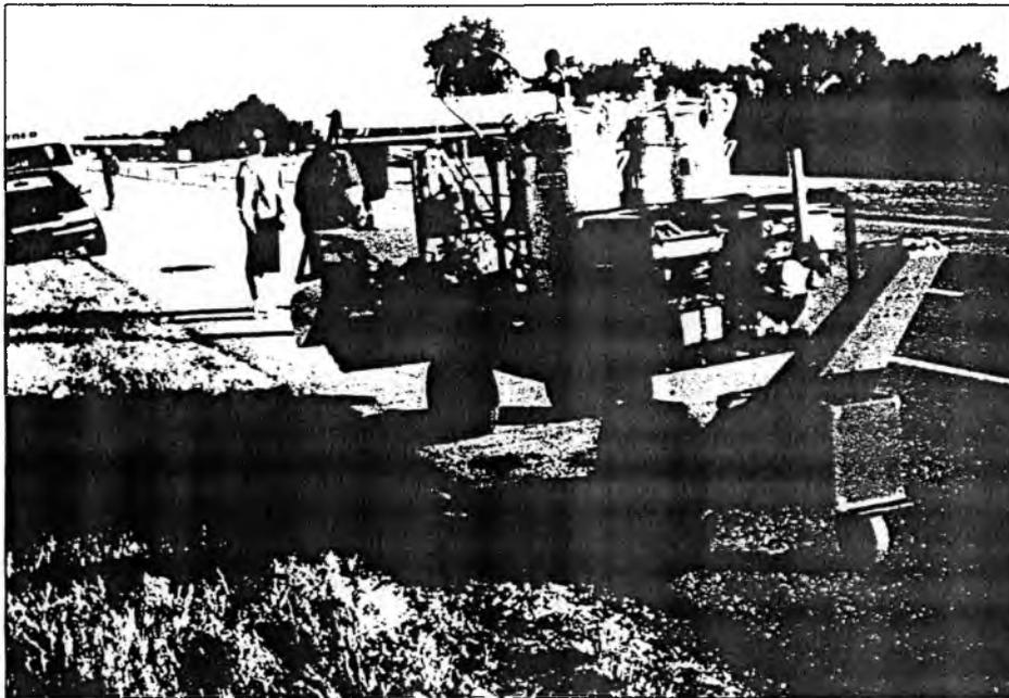
Convergent Spray Technology is applied in 4 hours as an anti-skid overlay on a bridge deck on Interstate 65 south of Huntsville.
