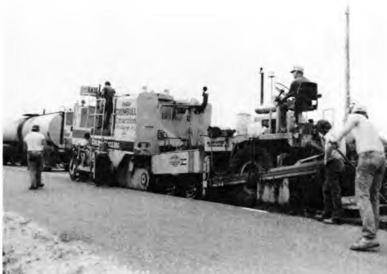
*Figure 3. The supply trucks, recycling machine and paver work closely together in a recycling train.*
