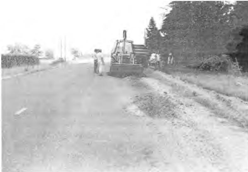
*Figure 4. Patching one of the worst deteriorated areas before placing binder and surface.*
