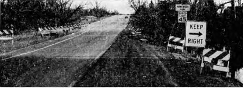
Figure 2. Problem obvious—also shows need for continuous inspection and maintenance.
