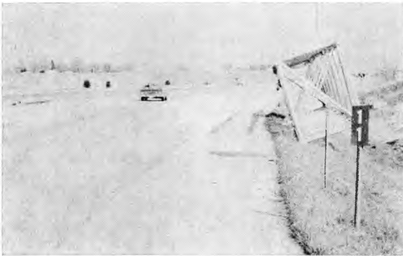
Figure 6. Obvious hazard—should be placed further from shoulder.
