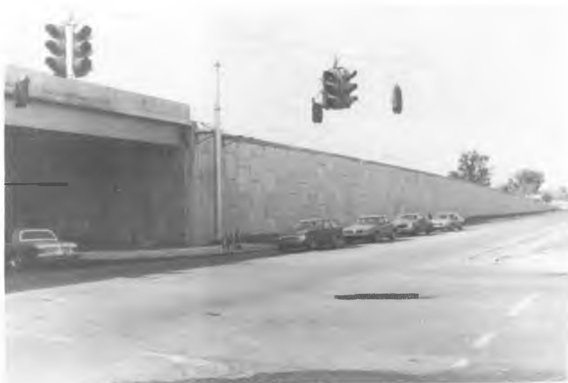
Typical Reinforced Earth™ structure. SR 66 Vanderburgh County (constructed by Traylor Brothers, Inc. and Industrial Contractors, Inc.)
