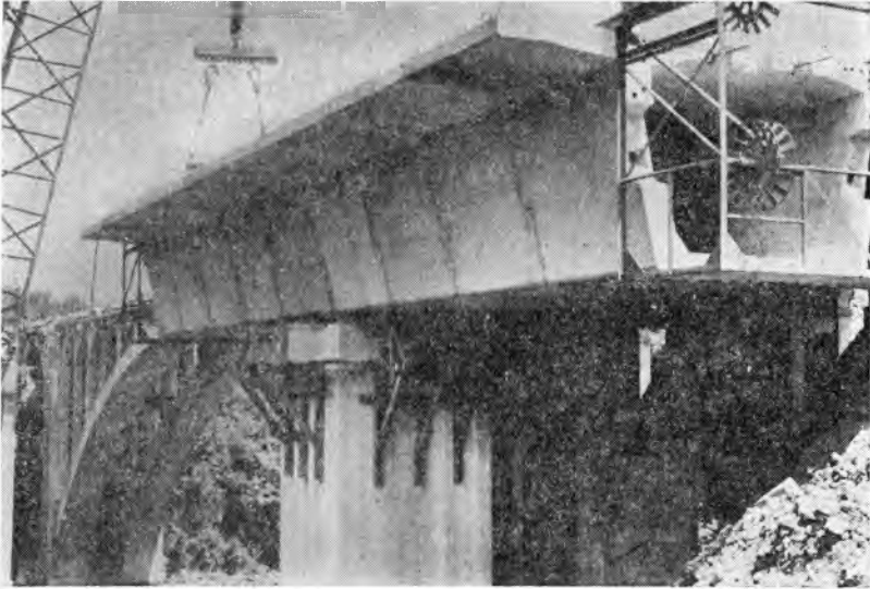
Figure 5. Here are nine segments balanced on a pier—there is a segment on the pier and four on each side. The open center portion may be used to carry utility pipes and wires and provides a walkway for inspections.
