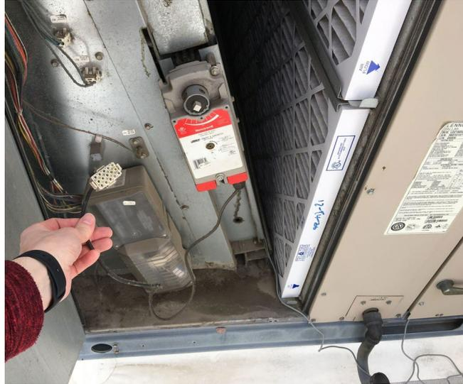
**Figure 2:** RTU economizer fault caused by disconnected actuator plug
