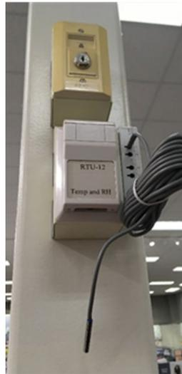
**Figure 1:** Data logger sensor beside the BAS's zone temperature and relative humidity sensor
