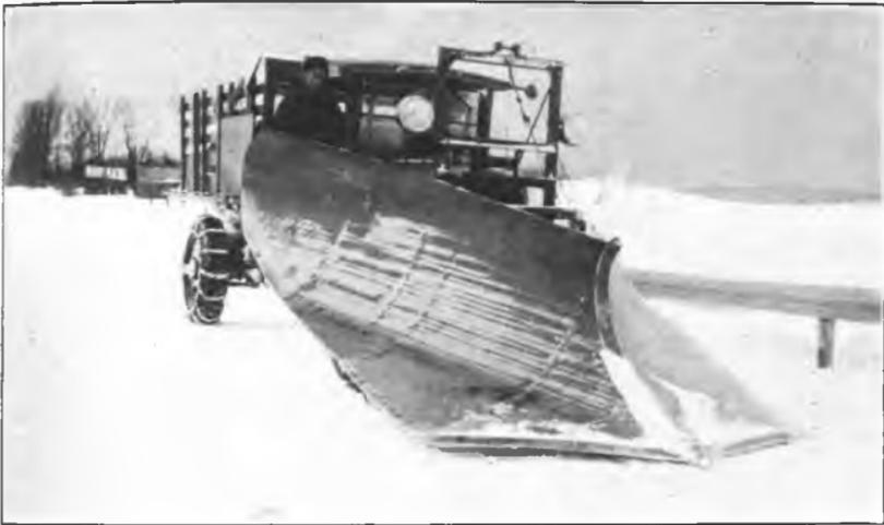
Fig. 3. "V" Shaped Snow Plow Attached to Truck.
