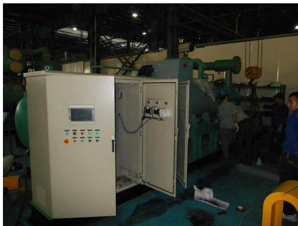
Figure 5: Generator and Synchronizing Equipment
