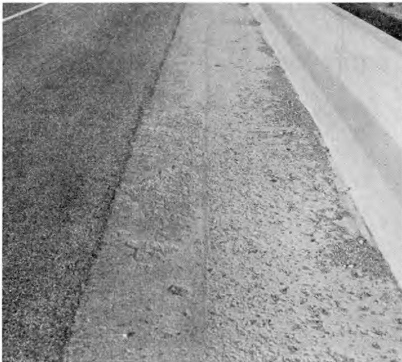
**Fig. 5.** A bridge deck scaling survey in 1964 found some scaling and other deterioration on bridge surfaces of recent construction. The season of construction and low air content were indicated as possible causes of failure.
