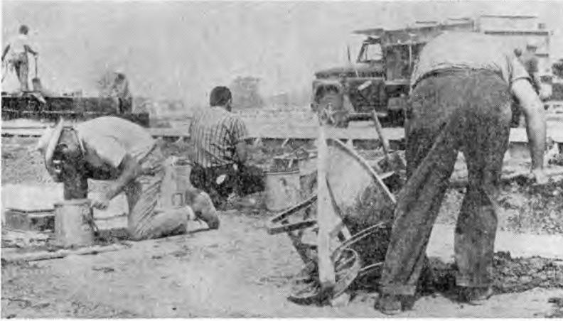
Fig. 6. A research project in the area of quality control of highway construction included field tests on concrete being placed for a new highway.
