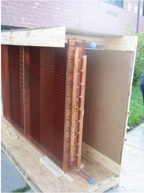
Figure 1: Copper heating coil, as delivered on site.
