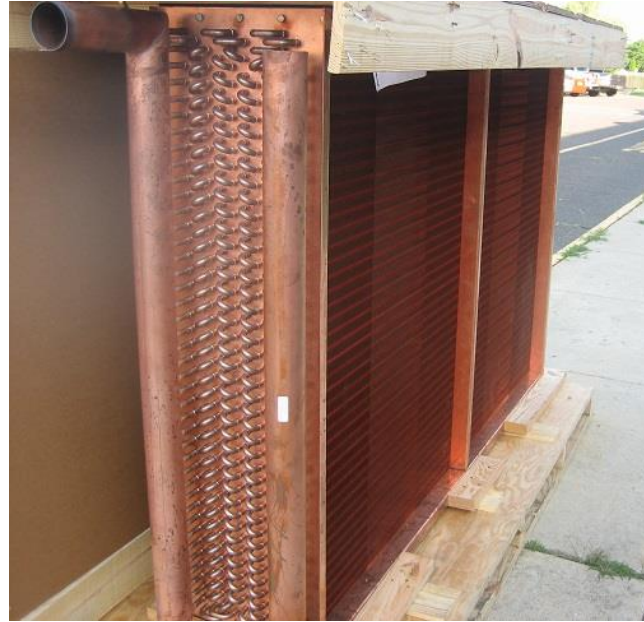
Figure 2: Copper cooling coil, as delivered on site.
