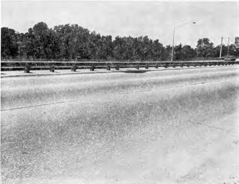
Figure 5. An asphaltic concrete pavement—gravel aggregate—after six winters of studded tire traffic—approximately 9,800 ADT per lane—estimated 1.0 million total studded tire passes.
