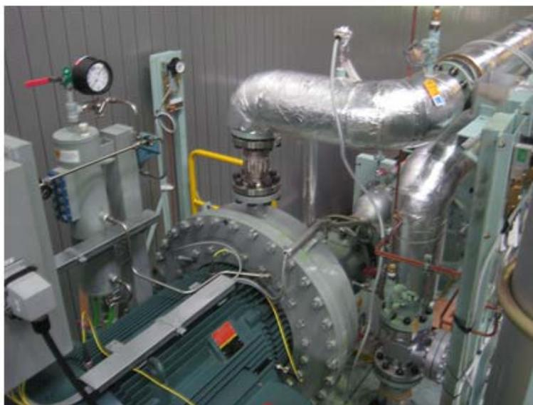
**Figure 5:** Two Hundred Kilowatt (200kW) Two-Phase Impulse Turbines Operating with R245fa
