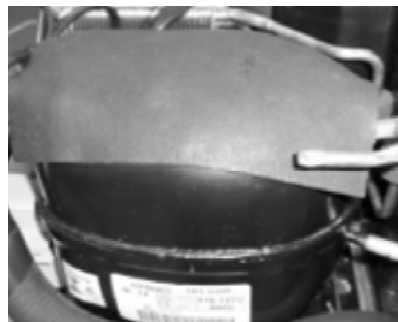
Figure 4: Position and size of asphalt blanket on compressor cover.
