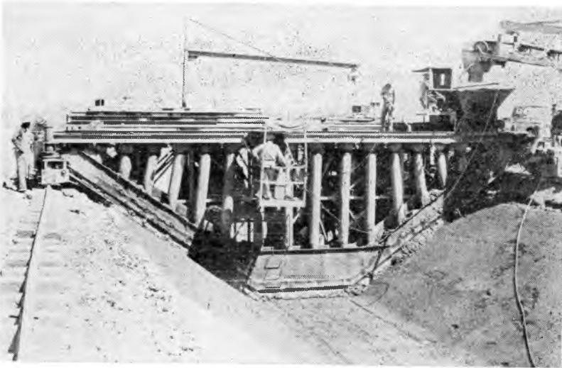
Fig. 9. Slip-form used in placing three-in. thick concrete lining of large canal. Concrete must be on dry side to prevent sloughing on side slopes.
