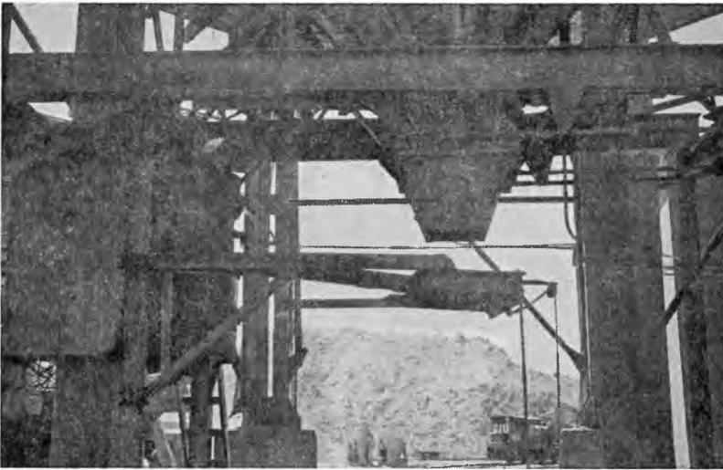
Fig. 12. Sampling tray which is swung under concrete hopper to obtain two cubic feet of concrete for tests.
