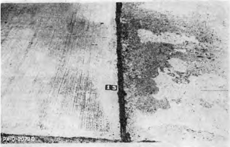
Fig. 3. Superior resistance of air-entrained concrete pavement to heavy and frequent applications of salt is demonstrated by the concrete on the left compared to the concrete at the right which was built similarly in all respects except that the pavement on the right contained no entrained air.
