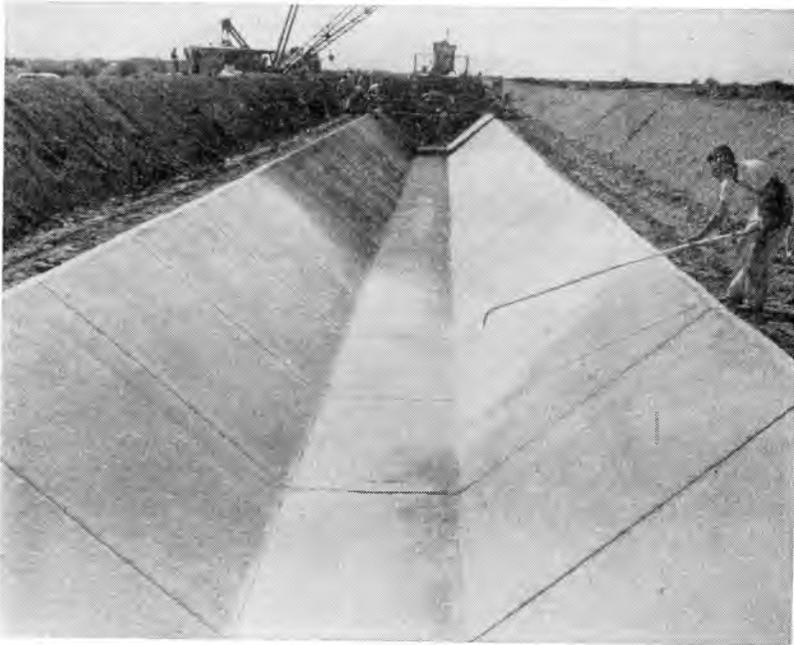
Fig. 10. Finished lining is cured with sealing compound immediately after finishing.
