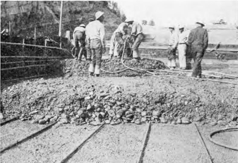
Fig. 7. Concrete at about one-in. slump containing aggregate graded up to six-in. in size is compacted in layers in Canyon Ferry Dam by heavy two-man internal vibrators. Concrete contained two sacks of portland cement and one sack of fly ash.
