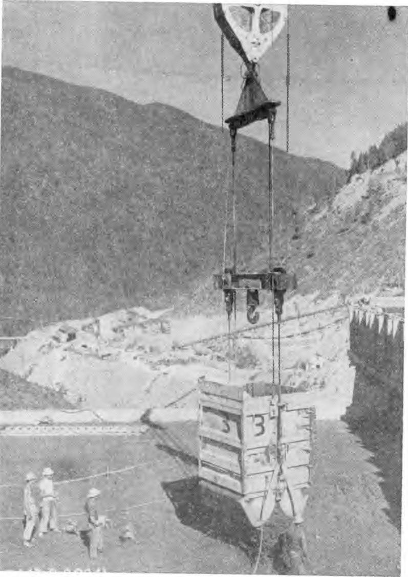
Fig. 6. An eight-cubic-yard bucket being emptied in block of Hungry Horse Dam. Transportation by highline and bucket usually causes little segregation. The eight-cubic-yard pile of concrete requires considerable work with large vibrators to consolidate into horizontal layers of not more than 20 in. deep.
