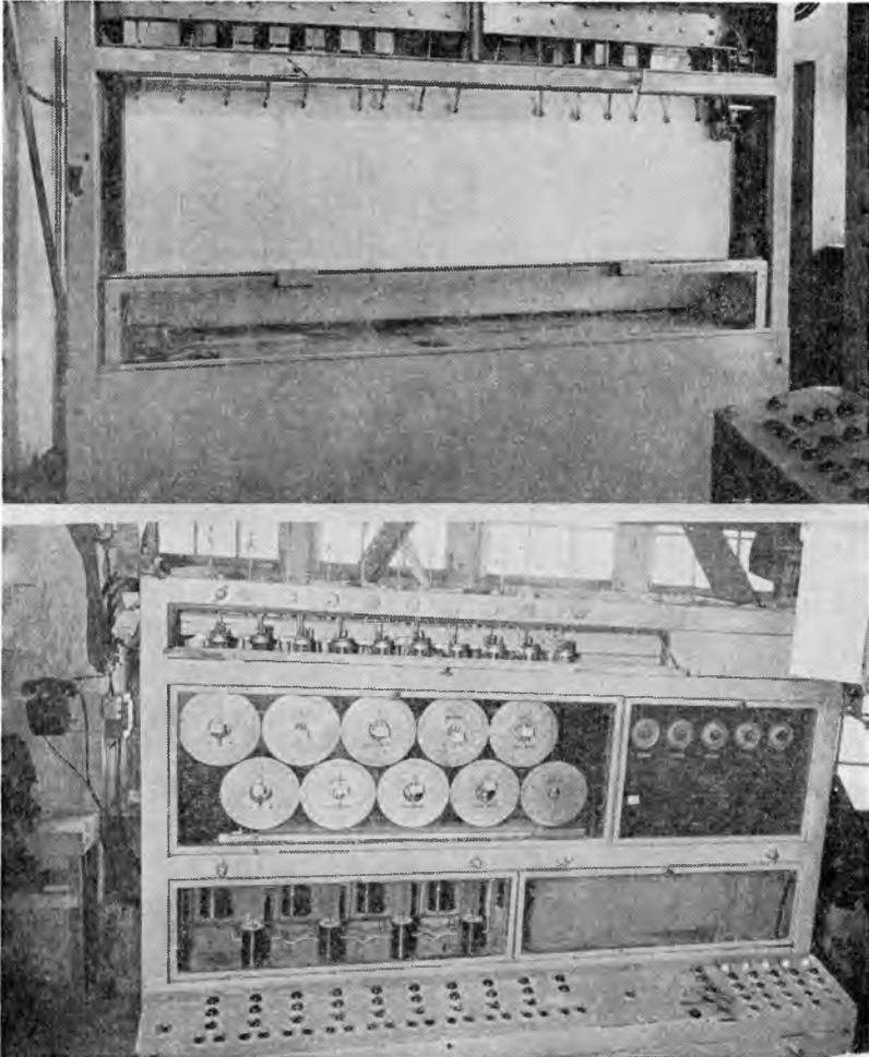
Fig. 5. Automatic batching control cabinet at bottom and recorder cabinet at top of picture used in construction of Hungry Horse Dam. Modern plants will automatically select, batch, and mix the proper proportions of as many as ten liquid, solid, powdered, or granular materials.
