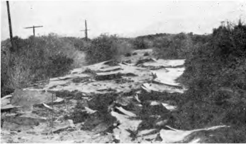
Fig. 1. Barrack floor failure a few years after construction from sulfate attack.
