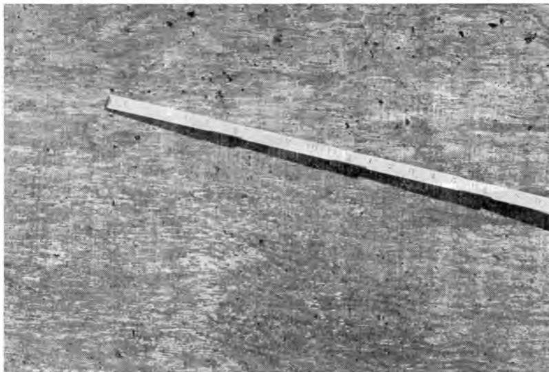
Fig. 8a. Bug holes which were removed by vibration as in Fig. 8.
