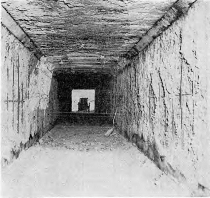
Fig. 11. Culvert destroyed by fire resulting from burning of wooden forms which were ignited by heater used to protect concrete from freezing.
