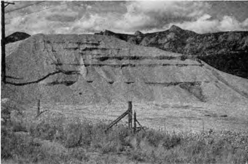
Fig. 4. This stockpile of processed aggregate was built in layers by trucking over each layer. The trucks caused breakage and contamination. Amount of undersize varied, sometimes running as high as 30 per cent.
