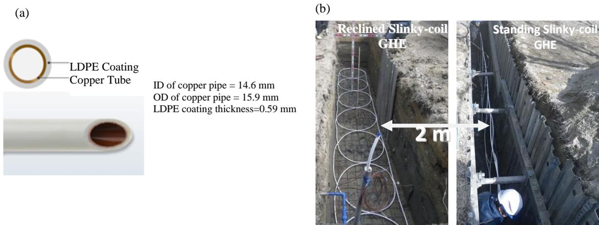
**Figure 1:** (a) Outer surface LDPE coated copper tube, (b) Installation of slinky-coil ground heat exchangers
