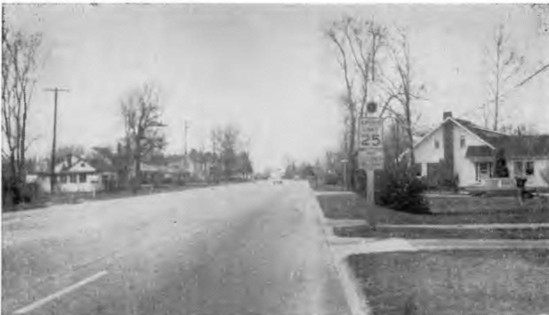
Fig. 4. Traffic control device used—special speed limit sign with single flashing signal.
