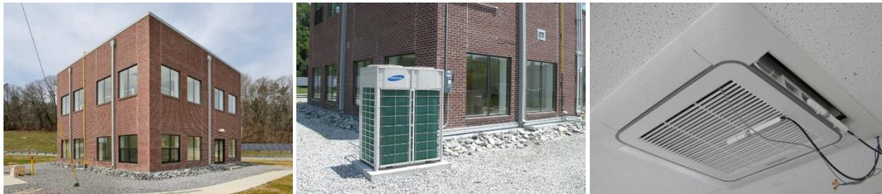
**Figure 1:** Test facility (1a-left), VRF system's outdoor unit (1b-center) and indoor unit (1c-right)
