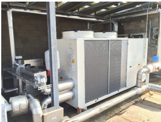
Figure 7: A/W Chiller Equipped with Variable Speed Scroll Solution (left) and test results (right)
