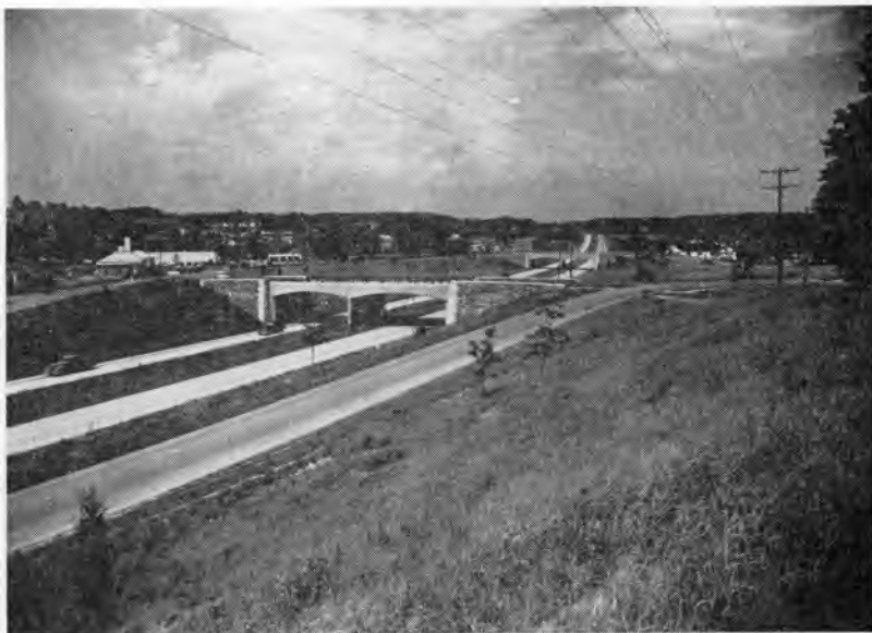
Fig. 2. Rotary intersection at junction of the Shirley Memorial Highway, Seminary Road and Gunston Road, Virginia. Through traffic flows freely on this expressway that provides access to housing developments and shopping areas.
