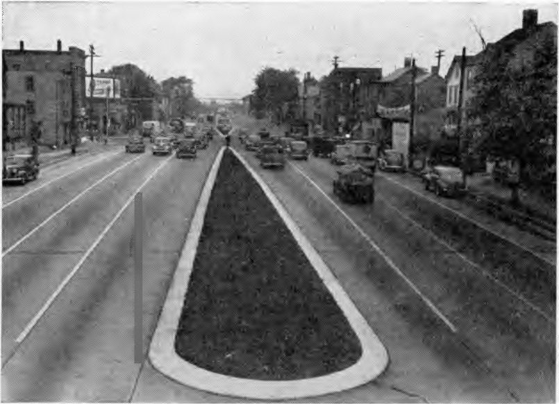
Fig. 1. U. S. Highway 1 at Elizabeth, New Jersey. Because the margins of this facility are not protected the functional service of the highway is reduced.
