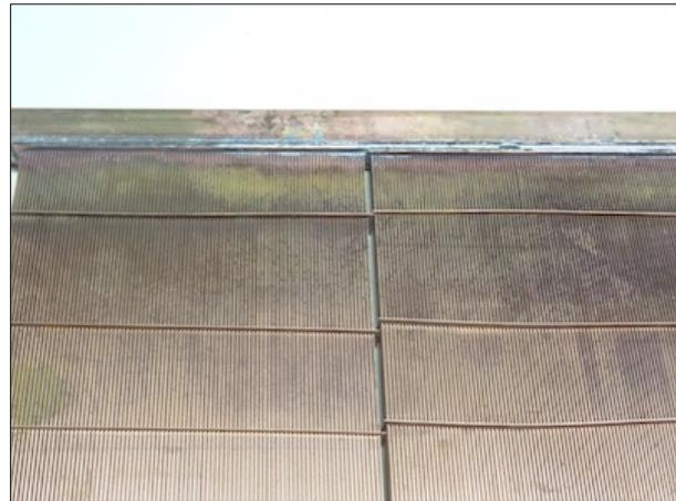
**Figure 8:** Outer spacer used as header – soldered to square manifold
