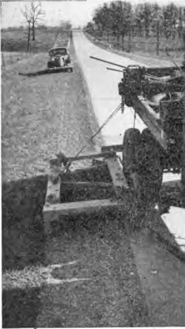
Left—Berm drag without roller, used excepting in spring.
