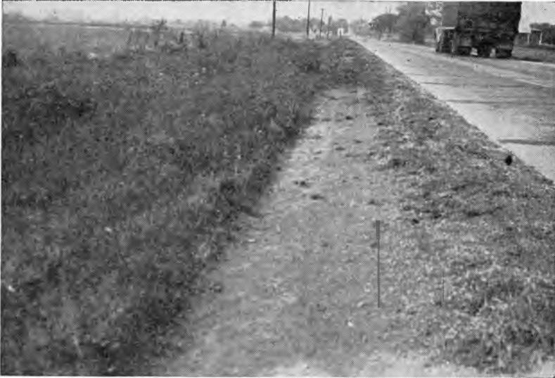
"Making" berm material by using a grader and creating a "false ditch." No use trying to seed here.
