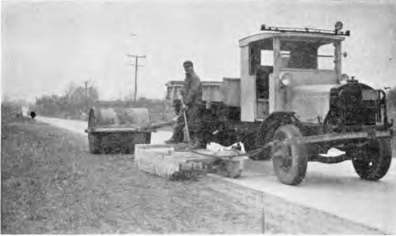
Berm drag and roller, used in spring. Roller is homemade. Weight—empty, 1,200 pounds; filled with sand, over 2,000 pounds.
