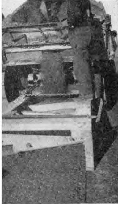
Right—Berm drag in operation. "Tailgating" extra berm fill material.
