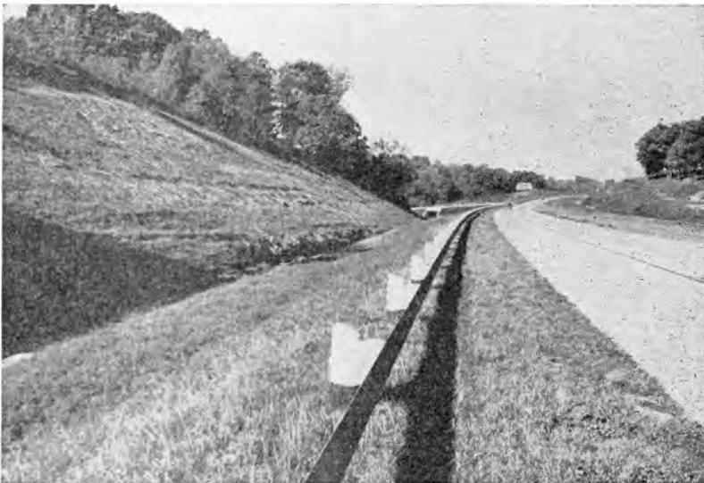
U. S. Route 40, Muskingum County, Ohio. Shoulders have been constructed to regular highway specifications and seeded. Shale slopes have been seeded and mulched. Constructed, 1943; photo, 1944.
