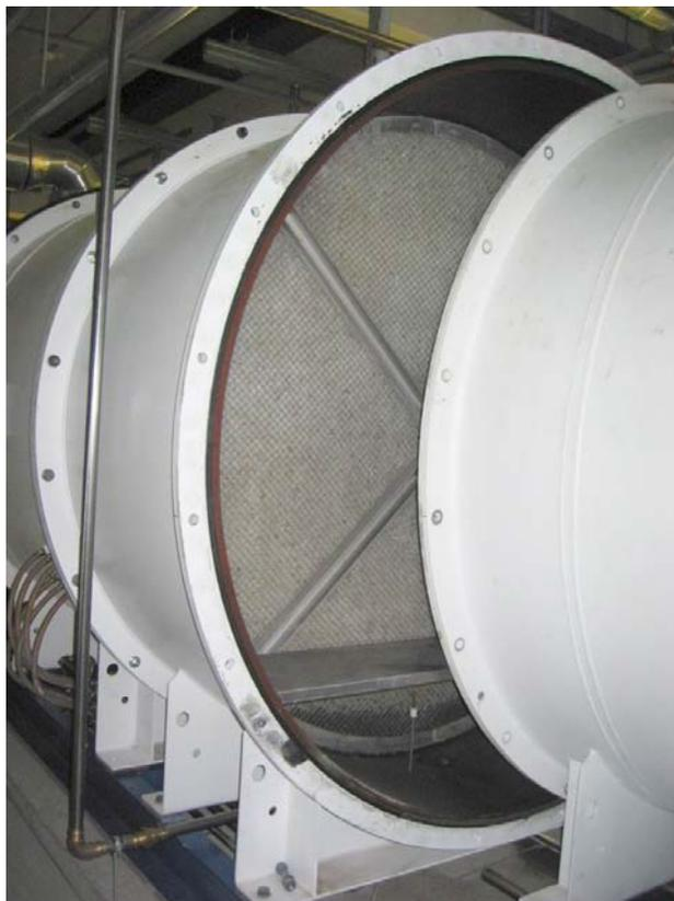
Figure 6: View of the opened intercooler
