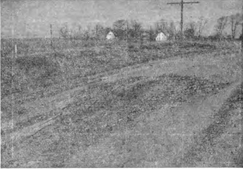
FIGURE 1. Failure of a flexible pavement in a shallow cut which intersects the plastic "B" horizon.
