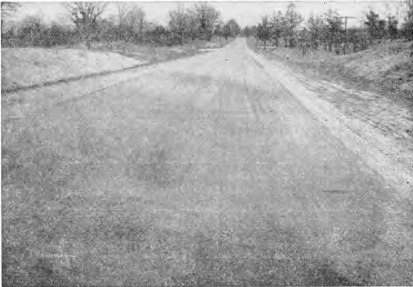
FIGURE 2. Good performance of a flexible pavement located on granular soil.
