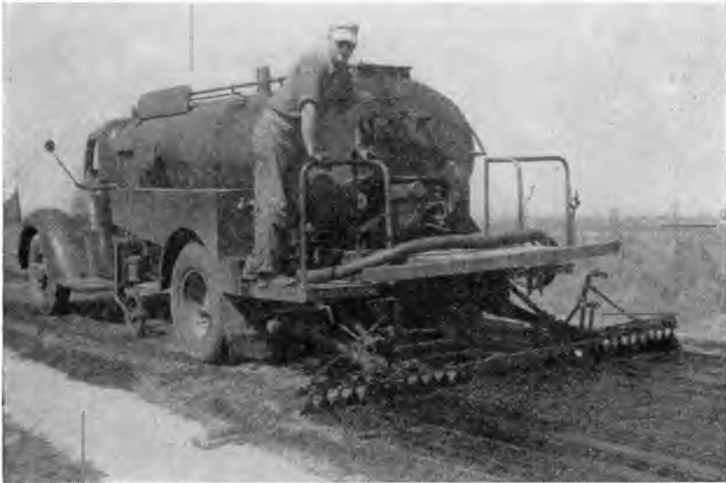
Applying bituminous material to aggregate.
