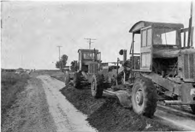
Road-mixing bituminous material and aggregate.
