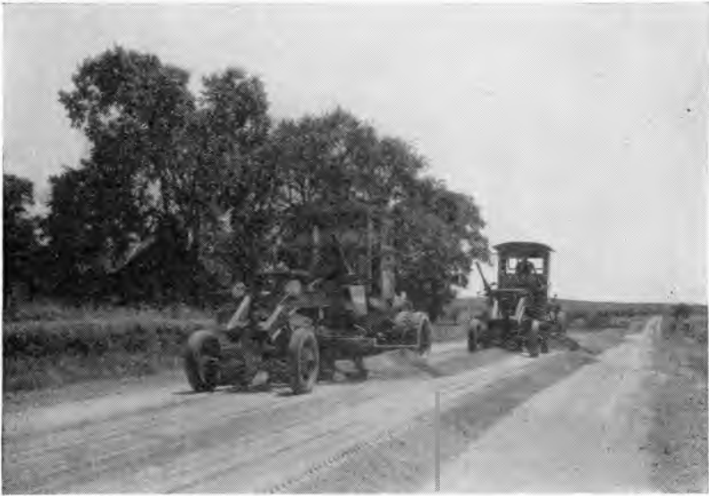
Drying aggregate before applying bituminous material.
