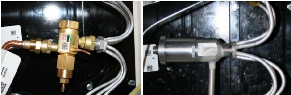
**Figure 2: Modified Thermostatic Expansion Valve With External Distributor And Integrated Valve and Distributor**
