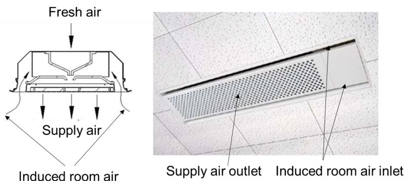
**Figure 1:** Schematic of induced-air supply unit (left) and the picture of unit after installation (right)
