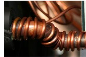
b) capillary tube externally attached
