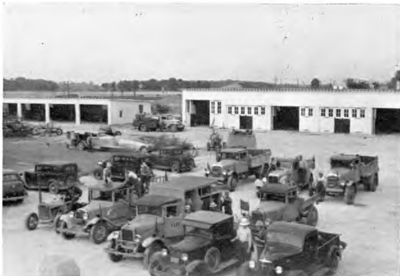
Many fail to realize the need of a great quantity of various types of equipment to maintain our highways. This is a view of some of the equipment and storage space at the Greenfield District headquarters.
