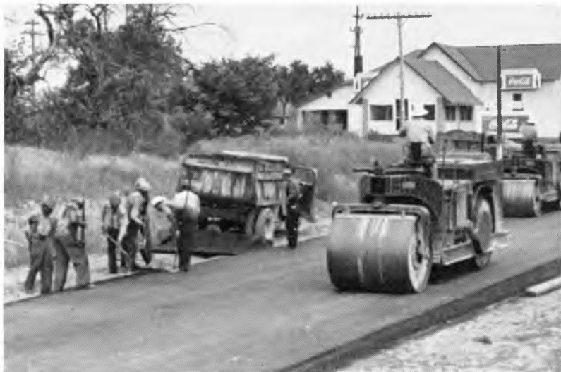
Bituminous resurfacing and widening strip at a highway intersection.
