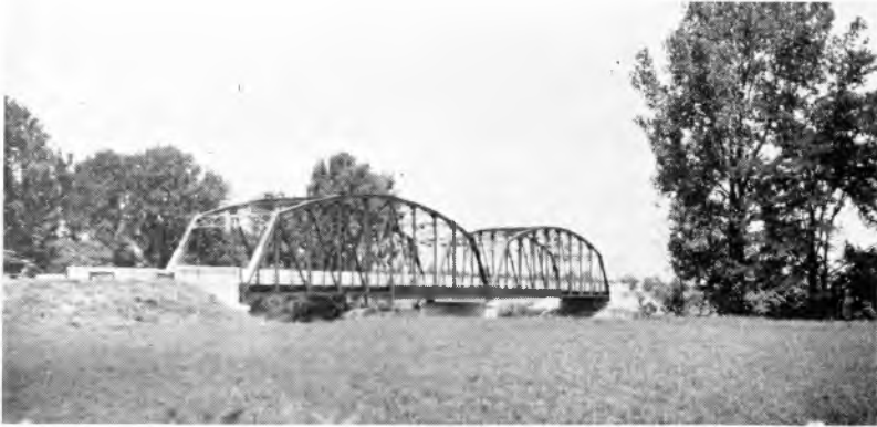
A typical stream-crossing of prewar days. With ample roadway clearance and load-carrying capacity, it should serve traffic in a satisfactory manner for many years if properly cleaned and repainted as required.
