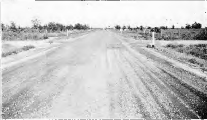
Fig. 2. View showing junction of stabilized and loose gravel sections on Michigan State Trunkline Road No. 20.
