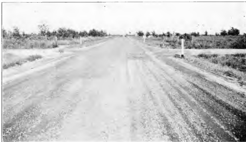
Fig. 2. View showing junction of stabilized and loose gravel sections on Michigan State Trunkline Road No. 20.
