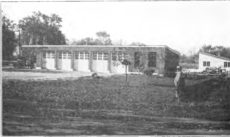
Fig. 1. Benton County garage with additional storage space in frame building at right.
