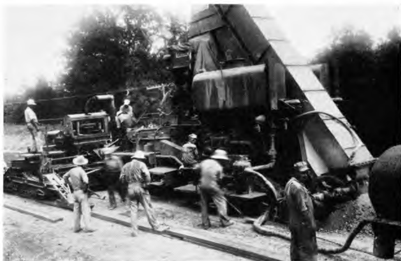
Fig. 1. Side view of Barber-Greene mixing machine and spreading unit.
