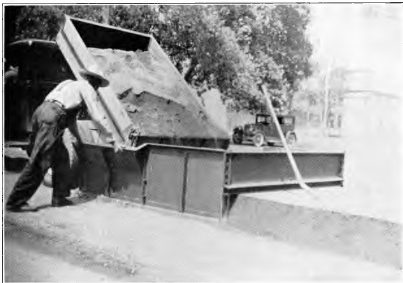
Fig. 2. Use of "Proportioner" in placing and measuring aggregate for road-mix.
