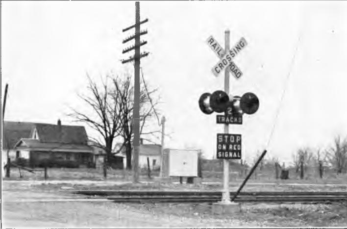
Fig. 11. Modern flasher signal. Notice reflectorized signs.
