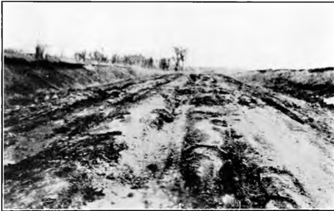
Fig. 1. A thin rubbery crust of dry material covering saturated unstable soil.
