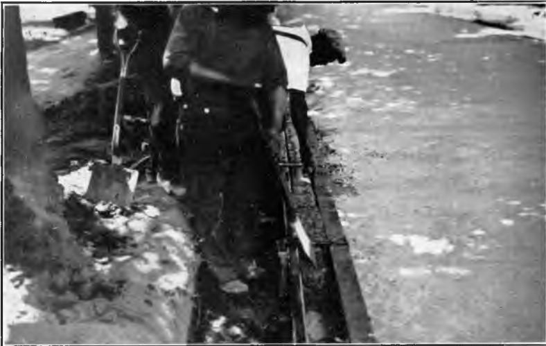
Fig. 6. Placing coarse aggregate in curb forms.
