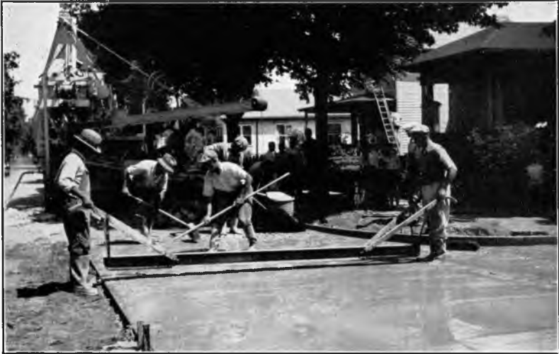
Fig. 3. Tamping after grouting.
