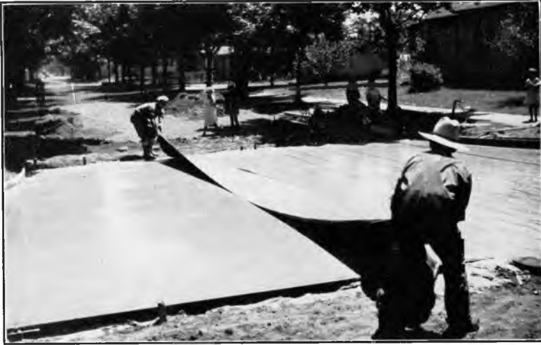
Fig. 5. Final finish with burlap drag.
