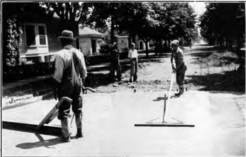
Fig. 4. Floating after grouting.
