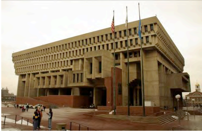
Figure 7: Kallman, McKinnel & Knowles, City Hall, Boston. Photo Alvaro Galve. Copyright release Creative Commons (CC BY-SA 2.0)
