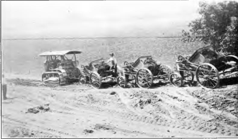
Fig. 1. Fulton County tractor and self-loading wheel scrapers grading a township road.
