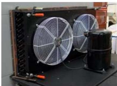
Figure 21: 5.0HP condensing unit
