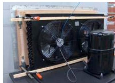
Figure 22: 3.5HP condensing unit
