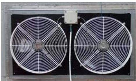
Figure 13: 450mm fans in parallel
