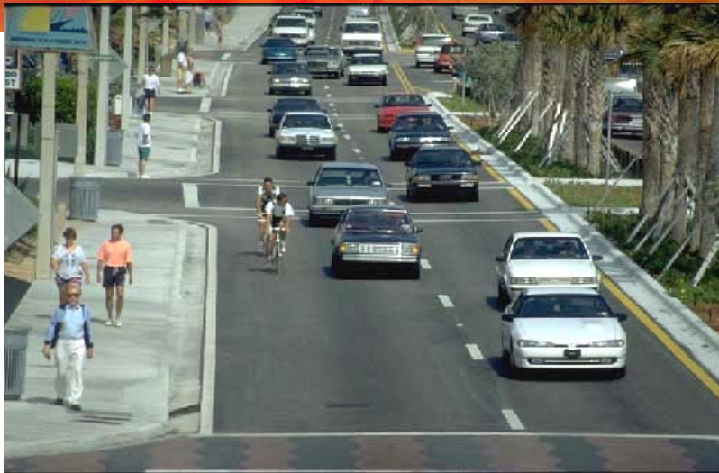
Example of a Wide Curb Lane
