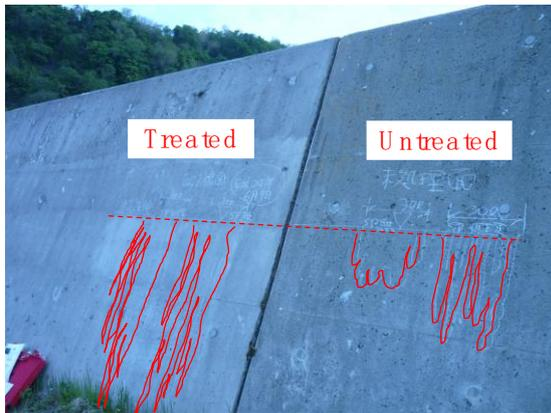
**Fig. 1** On-site situation —the effect durability of surface water repellency (watering test) (the 12<sup>th</sup> year)
