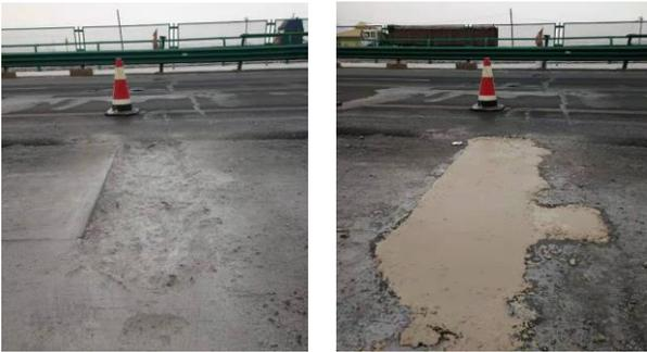
Figure 4. Magnesium phosphate cement rapid repair technology
