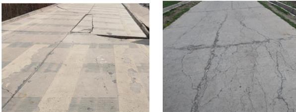
Figure 1. Broken slab of cement concrete pavement
