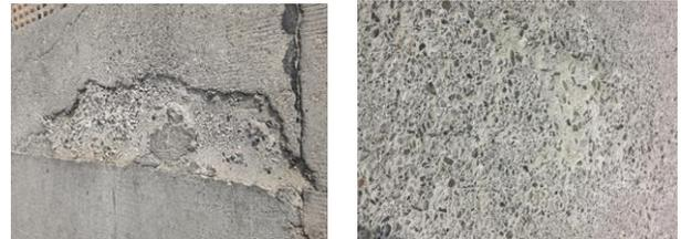
Figure 3. Surface diseases of cement concrete pavement
