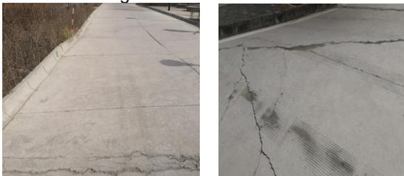
Figure 2. Cement concrete pavement subsidence
