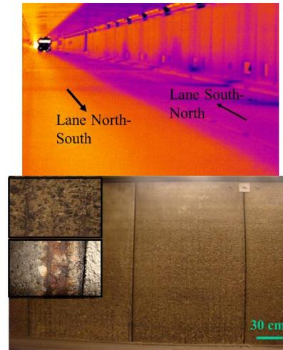
Fig. 2 Thermography and humidity distribution on the South entrance on the tunnel (left) and leaching as well as rebar corrosion of the wall panels (right).
