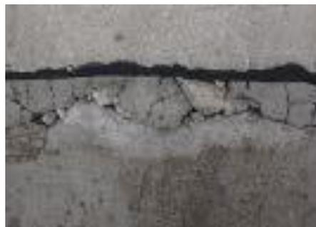
Figure 2. Edge breakage at expansion joint between the tunnel and the slab
